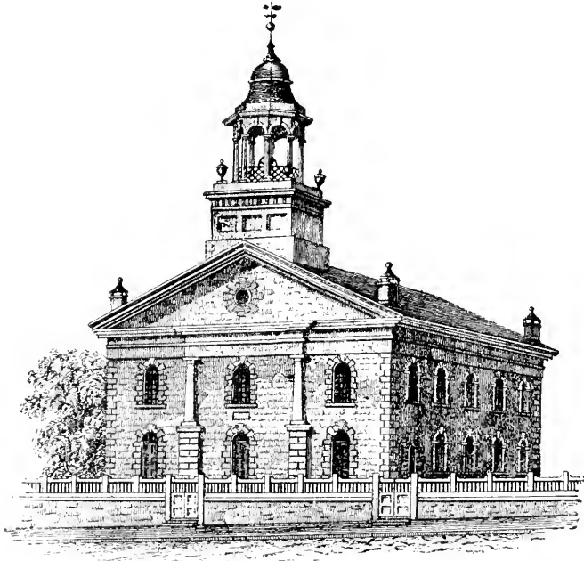
THE SECOND GARDEN STREET CHURCH, 1807 (SOUTH CHURCH)
